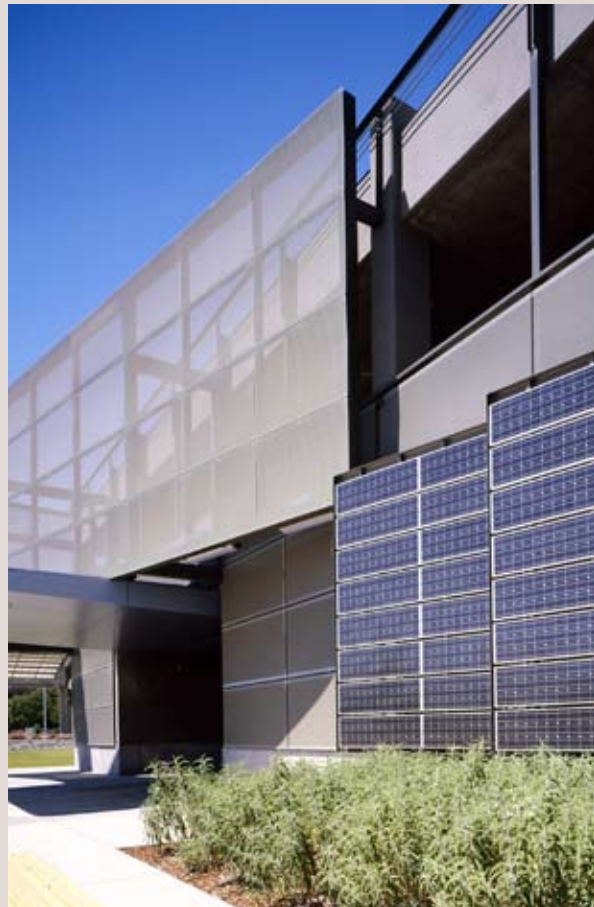
Solar panels adorn the side of the Fairfield Multi-Modal Transportation Center. © Stantec Architecture (formerly Chong Partners)
